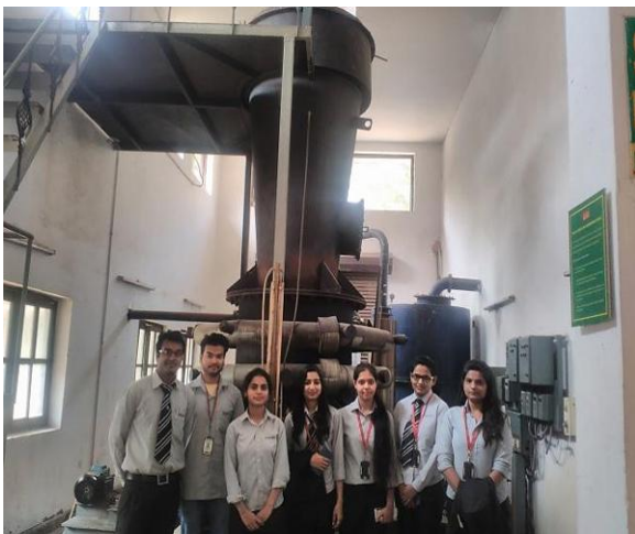
Students at Bomass Gasifier Room
